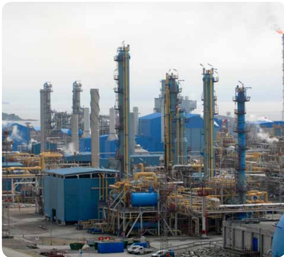
Fig. 5.1: Natural gas processing plant with gas/liquids separation columns, compressors, storage tanks etc. at Kårstø, Norway (Picture: Øivind Hagen/StatoilHydro).
